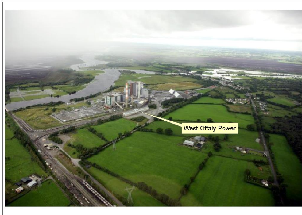
Figure 5-3 Aerial Photograph of the August 2008 Flood Event
